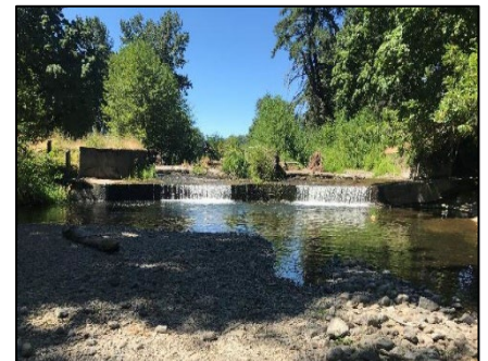
Balm Grove Dam on Gales Creek near Banks was permanently removed summer 2022 (statewide priority barrier).
