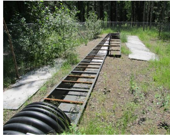
Large sediment loads in Sun Creek did not allow the fish screen to work properly.
