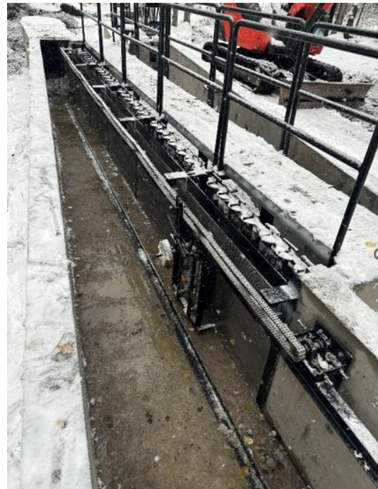
The new vertical flat panel screen is cleaned by a rotating brush powered by a paddle wheel.
