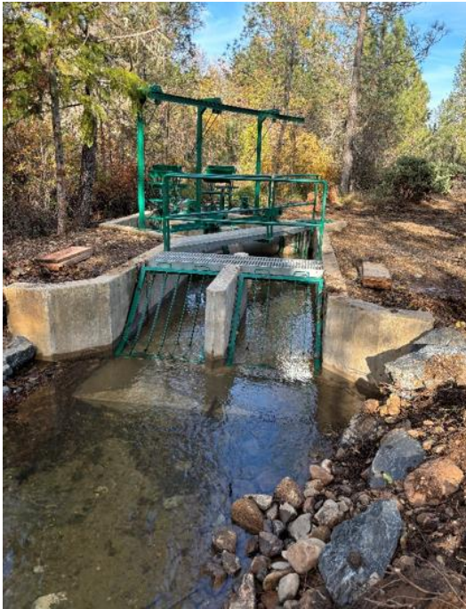
The new fish screen has a dual bay paddle wheel driven rotary drum.
