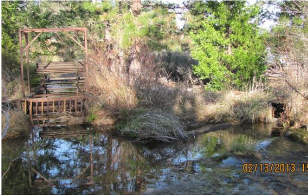
The old screen on the West Fork Illinois River was replaced in 2024.
