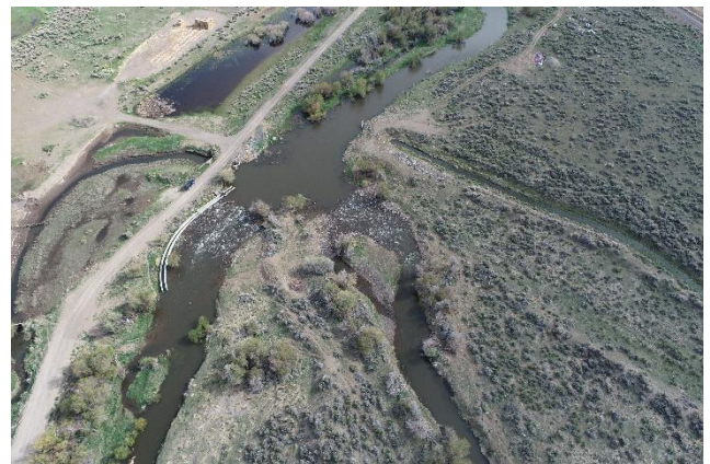
Looking upstream on Deep Creek at the Starveout Diversion. Two roughened riffles and sluiceway.
